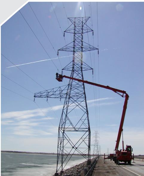
BSI monitors can be installed on energized lines, and will operate in all weather conditions. Research using the BSI demonstrated that it is as reliable as human observers for detecting collisions, and offers the advantage of providing continuous data recording even in the remotest locations. Data retrieval and changes to BSI settings can be performed remotely.
