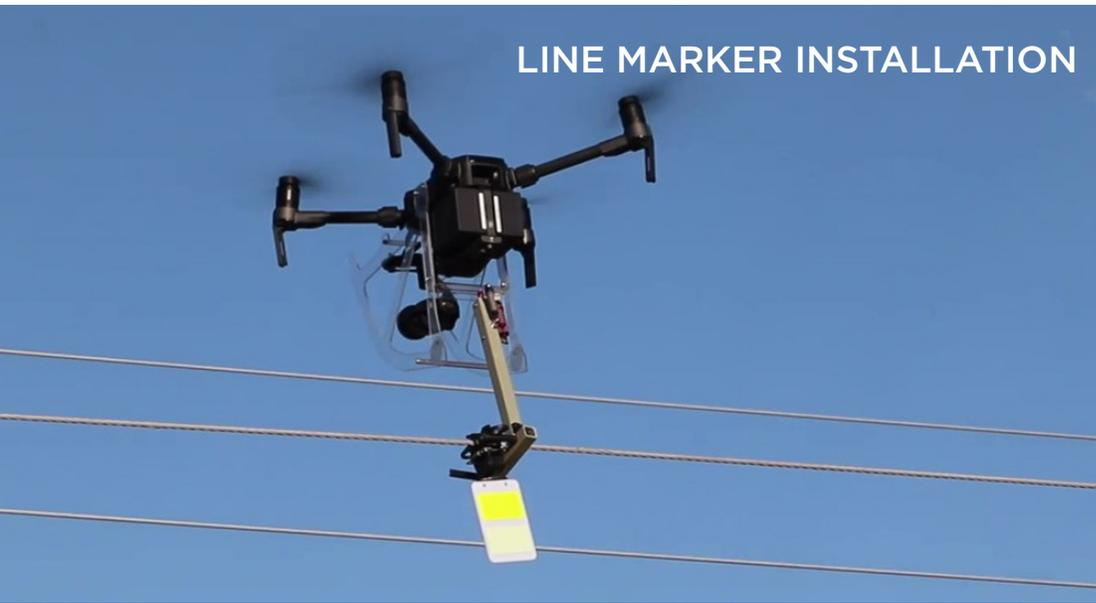
Line markers prevent collisions from both migratory birds and low-flying aircraft. Installation through EDM's proprietary UAS-mounted system saves time and money, and is far safer than helicopter installation.
